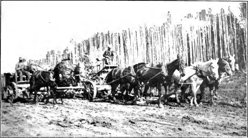
A grader at work on the right-of-way of the G.T.P.
